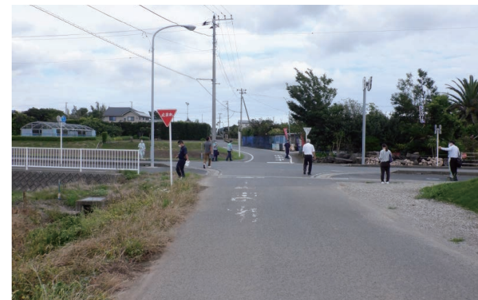
Before improvement: The "STOP" marking was fading.
