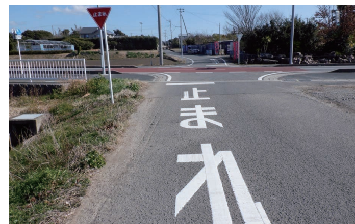
After improvement: The "STOP" line and letters were repainted and colored pavement within the intersection were added.
