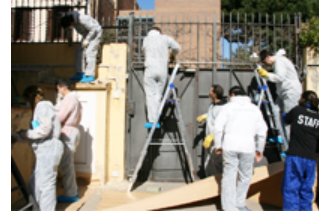
Associates make repairs at a children's home.
