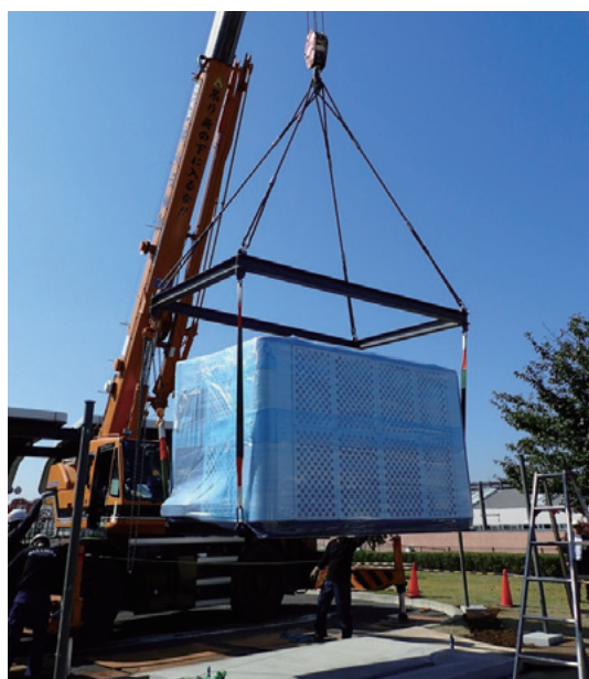
Fig. 5 Installation of SHS
