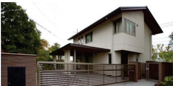
Fig. 2 Northwest side appearance of experimental house
