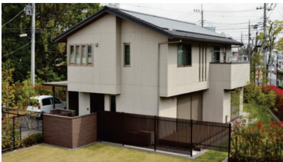
Fig. 1 Southwest side appearance of experimental house
