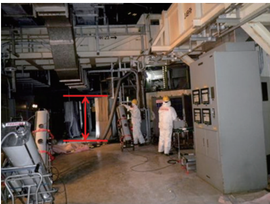
Fig. 4 Inside reactor building (Image provided by TEPCO)
