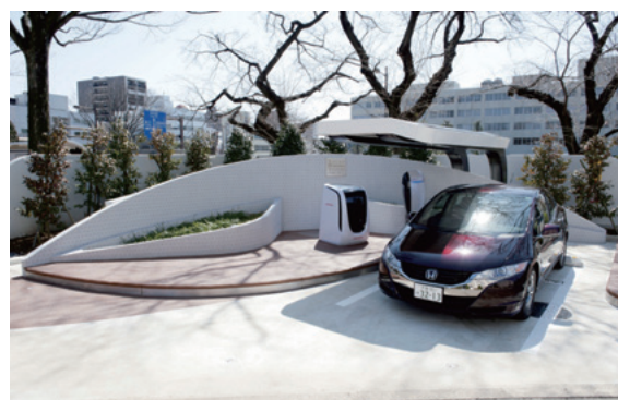
Fig. 2 External view of SHS2 installed on Saitama prefecture property
