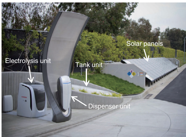
Fig. 1 External view of Solar Hydrogen Station (SHS2)
