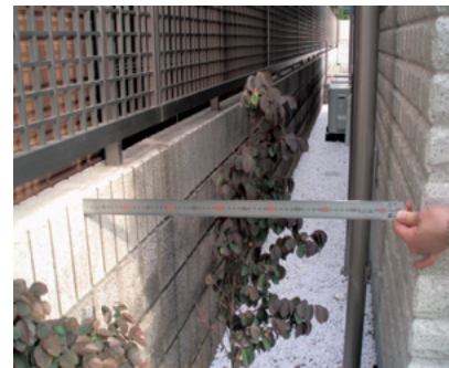
Fig. 2 Example of 650 mm exterior space
