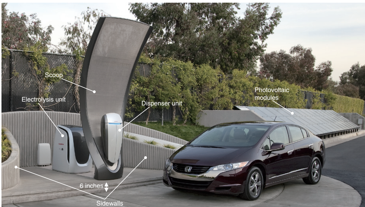
Fig. 1 External view of high differential pressure water electrolysis-type Solar Hydrogen Station (SHS2)
