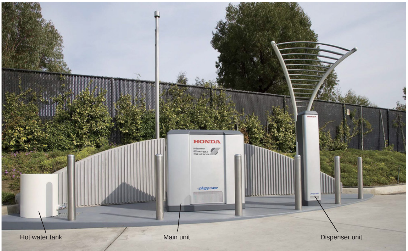
Fig. 1 External view of Home Energy Station IV
