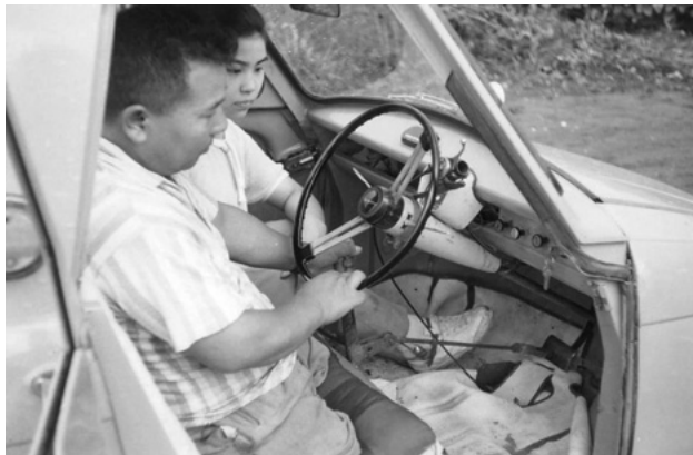
Fig. 1 Manually operated auxiliary driving device
