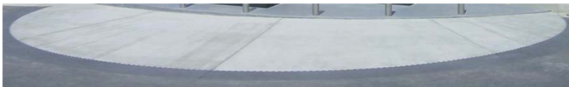
Fig. 11 Concrete fueling pad surface in front of hydrogen station
