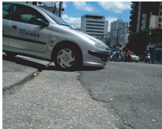
(d) Road surface at a drainage ditch in intersection
