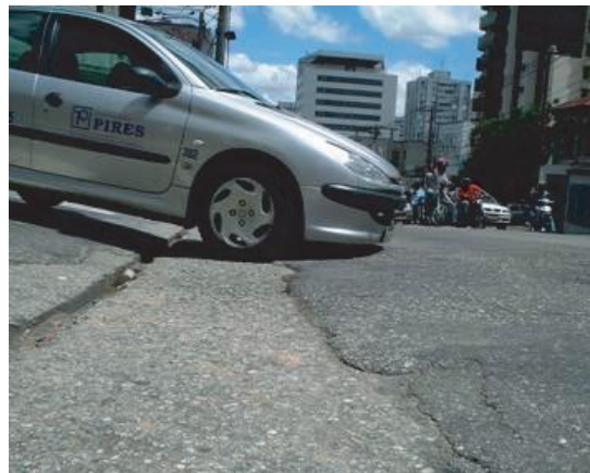
(d) Road surface at a drainage ditch in intersection
