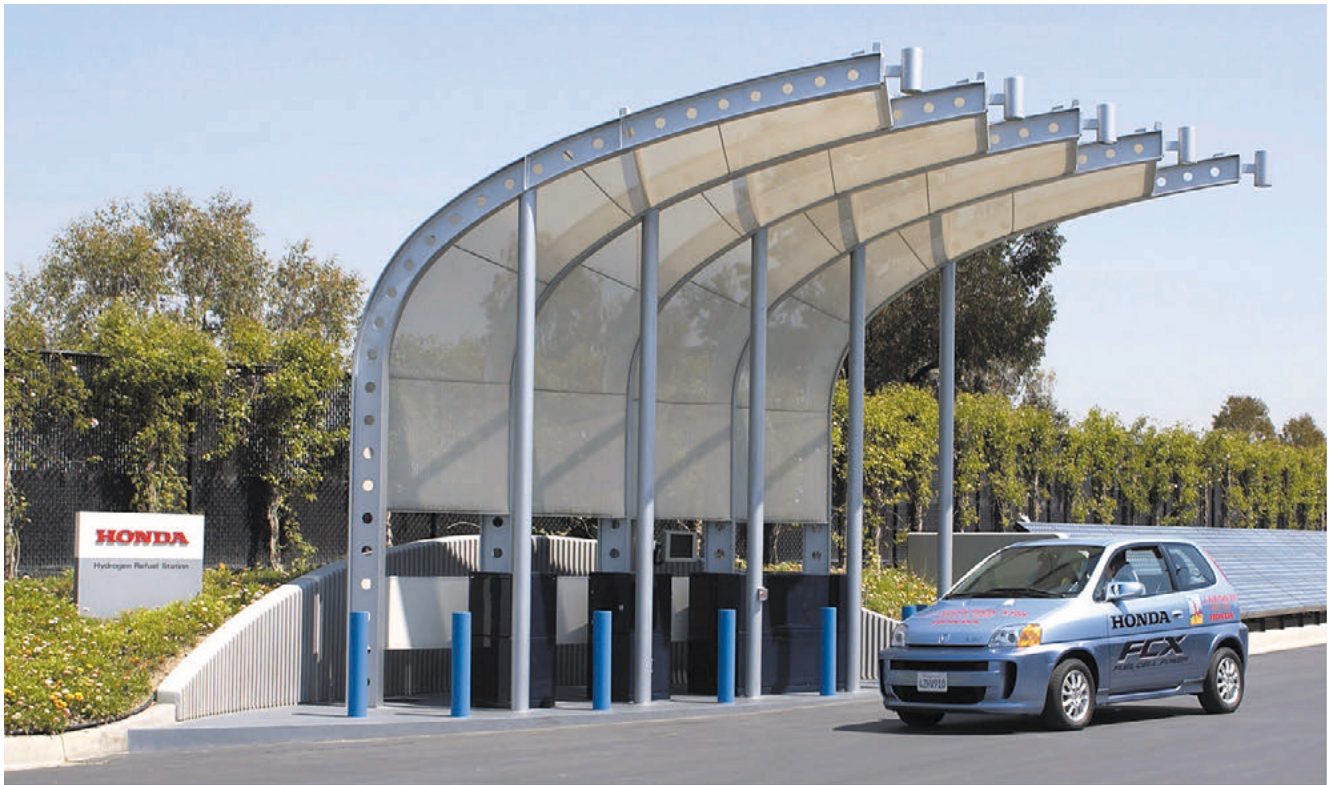
Fig. 1 External view of Hydrogen Refueling Station
