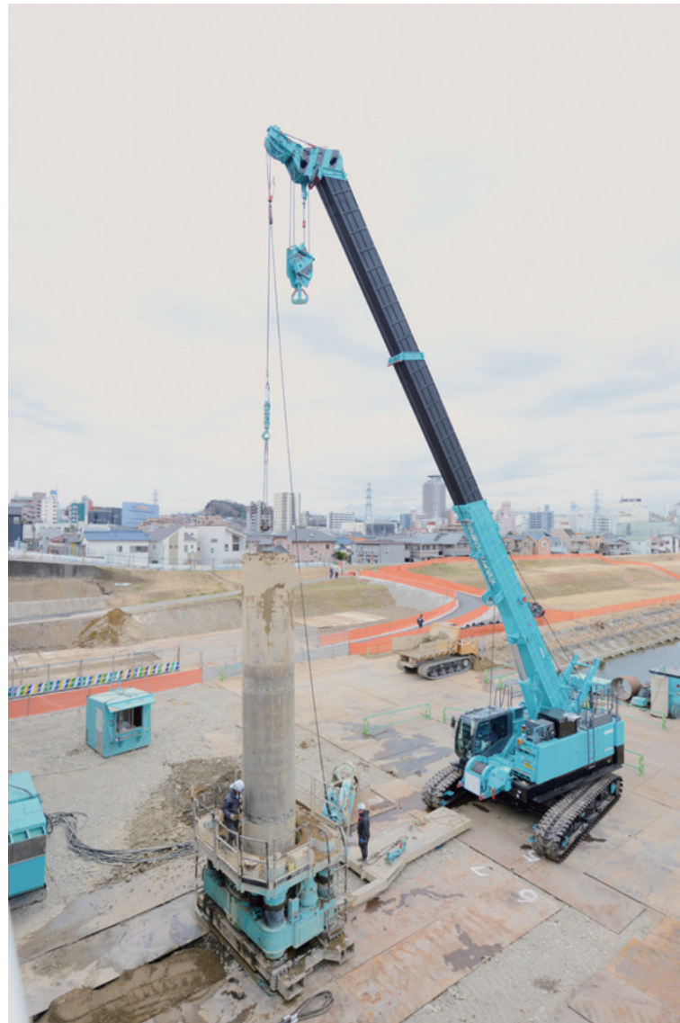
Fig. 6 Example of mobile crane (photo provided by KOBELCO Construction Machinery Co., Ltd.)
