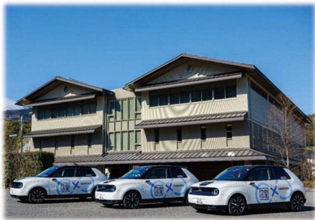
Fig. 5 Suzuhiro office building and EVs used for test
