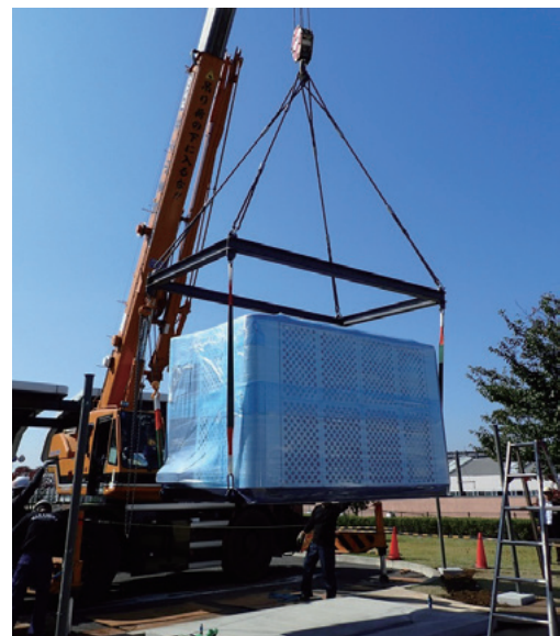
Fig. 5 Installation of SHS
