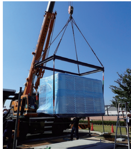
Fig. 5 Installation of SHS
