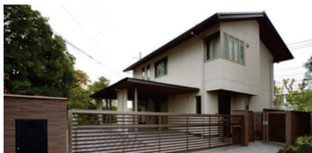
Fig. 2 Northwest side appearance of experimental house
