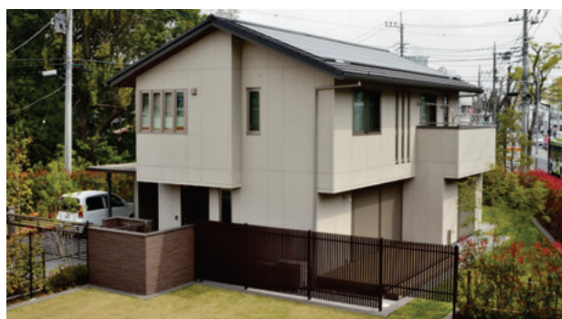
Fig. 1 Southwest side appearance of experimental house
