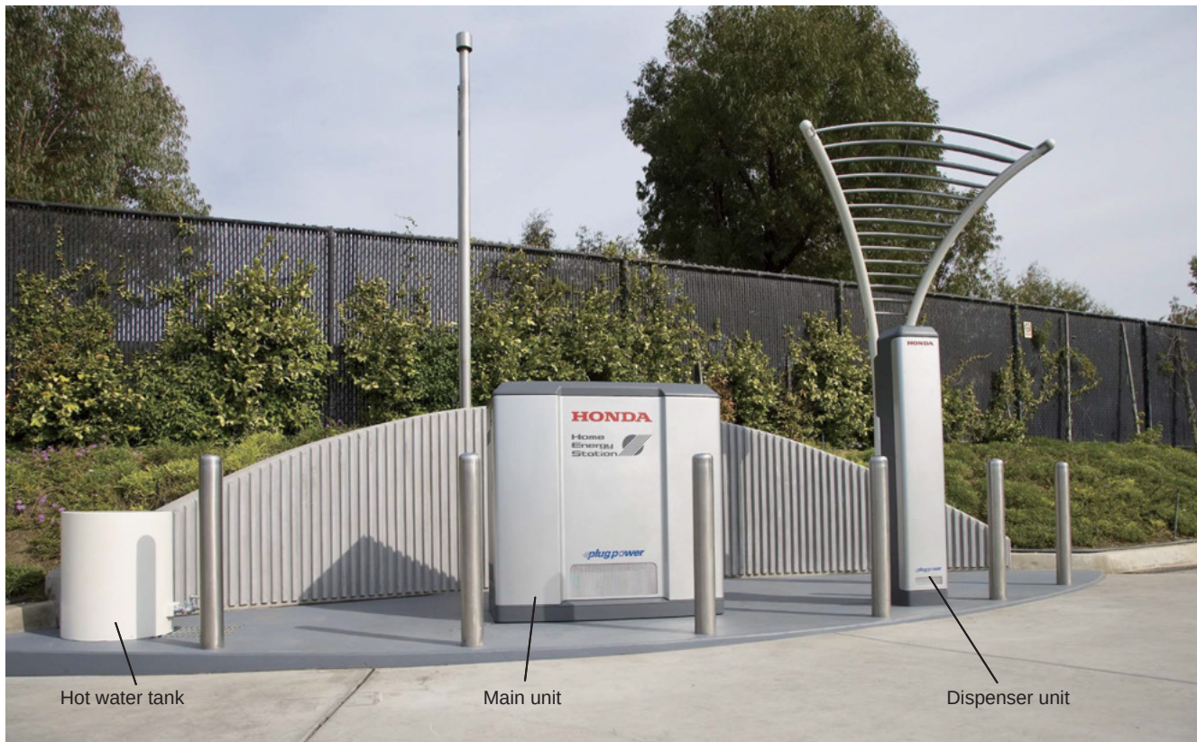
Fig. 1 External view of Home Energy Station IV
