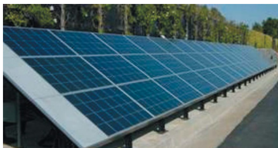
Fig. 2 CIGS thin-film photovoltaic modules (prototype; manufactured by Honda Engineering Co.,Ltd.)
