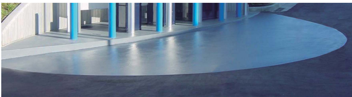
Fig. 10 Conductive paint fueling pad surface in front of hydrogen station
