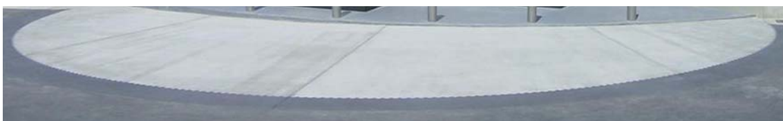
Fig. 11 Concrete fueling pad surface in front of hydrogen station
