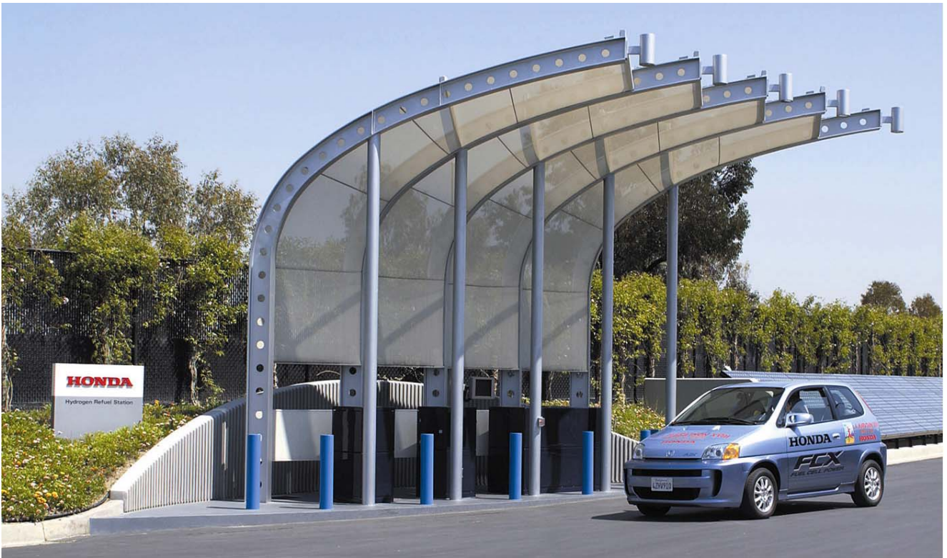
Fig. 1 External view of Hydrogen Refueling Station
