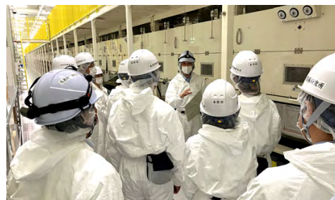
Honda R&D Co., Ltd. (Sakura) Inspection of the demonstration production line for all-solid-state batteries
