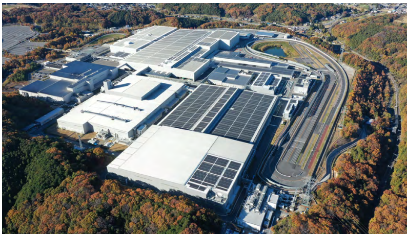
Saitama Factory Automobile Plant
