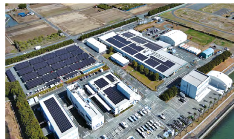
Hosoe Outboard Engine Plant (Japan)
