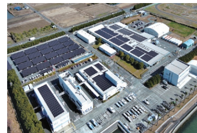
Hosoe Outboard Engine Plant (1.7 MW)
