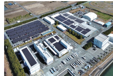
Hosoe Outboard Engine Plant (1.7 MW)
