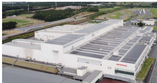
Kumamoto Factory (3.8 MW)
