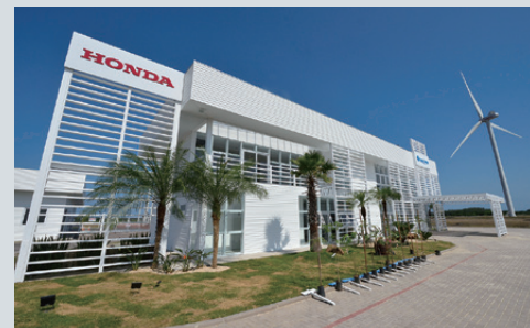
Honda Energy do Brasil Ltda., equipped with 9 wind power turbine units
