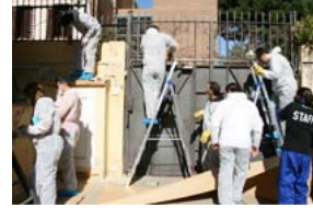
Associates making repairs at a children's home
