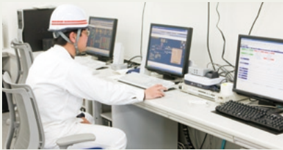
Monitoring using a system that manages energy consumption
