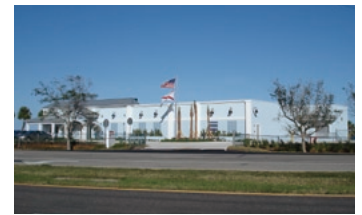
The marine outboard engines research facility in Florida achieved LEED Gold certification.
