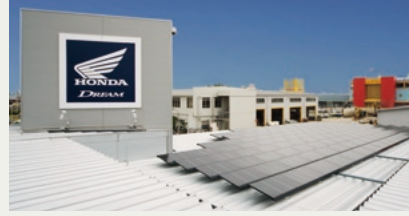
A total of 140 solar panel modules manufactured by Honda Soltec Co., Ltd., have been installed on the roof of Honda DREAM Matsusaka, providing 16 kilowatts of generating capacity. The system is expected to generate about 17 megawatt-hours per year.
