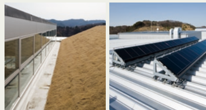
Rooftop greenification and solar panels
