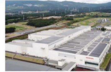
Kumamoto Factory (5.35 MW)
