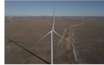
Bolling Springs Wind Farm (120 MW)
