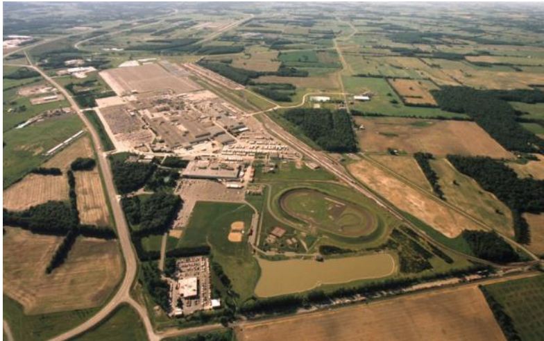
Marysville Auto Plant
