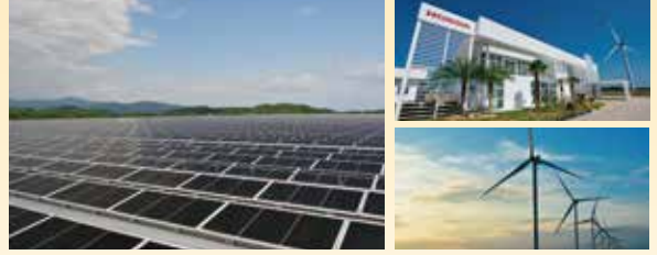
Honda Yorii Mega-Solar Power Plant (Japan)
