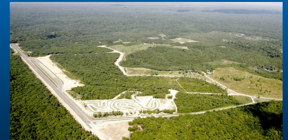
Manaus Plant (Brazil)
